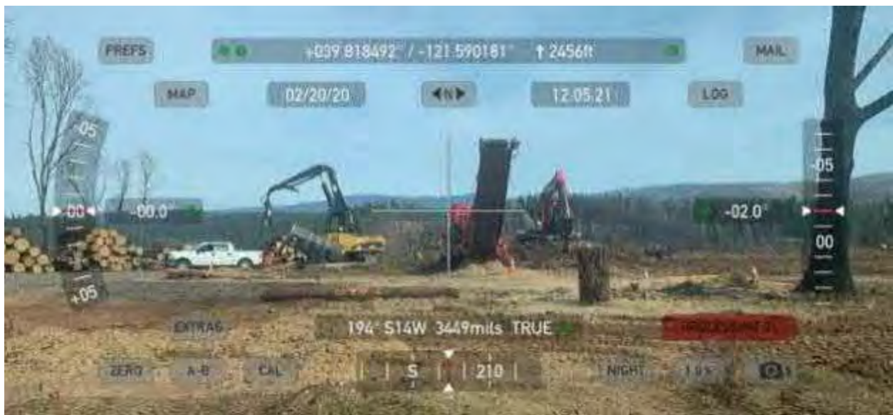
Photo 11. Tree removal equipment in use near Lake Ridge Circle. Paradise, CA.
