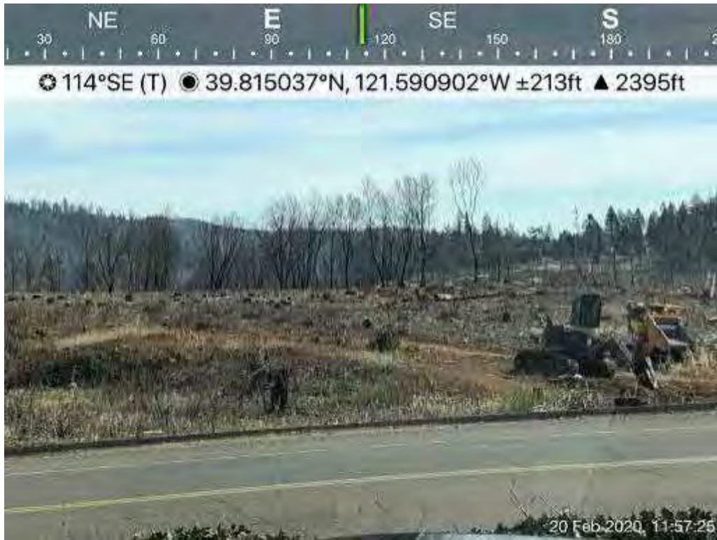
Photo 8. Partially completed tree removal near Pentz Road. Paradise, CA.
