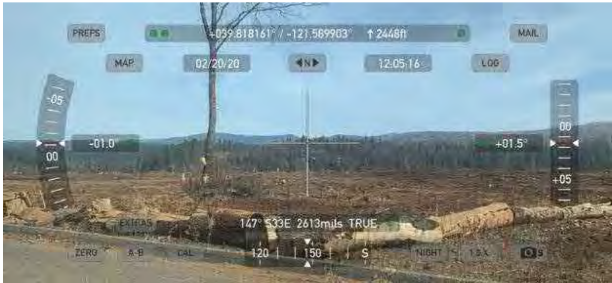
Photo 10. Completed tree removal near Lake Ridge Circle. Paradise, CA.
