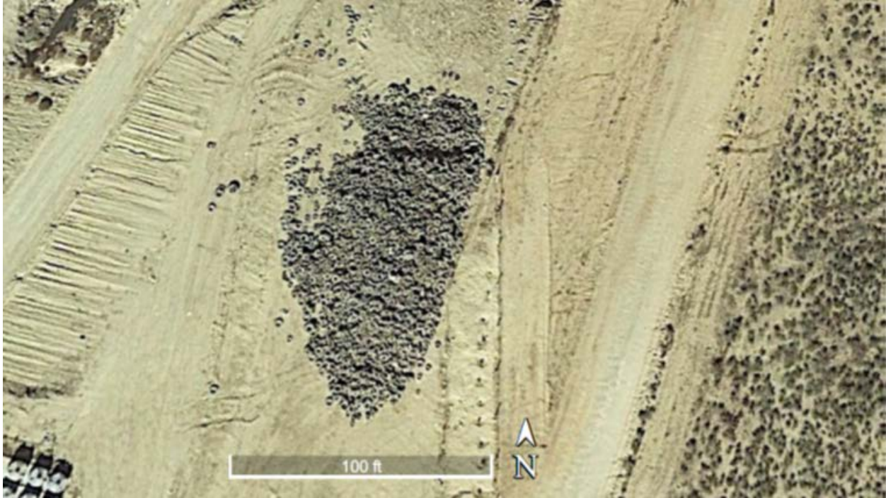
Image 16. Accumulation of waste tires at the municipal landfill of Playas de Rosarito, operated by GEN. November 2016. Source: GoogleEarth.
