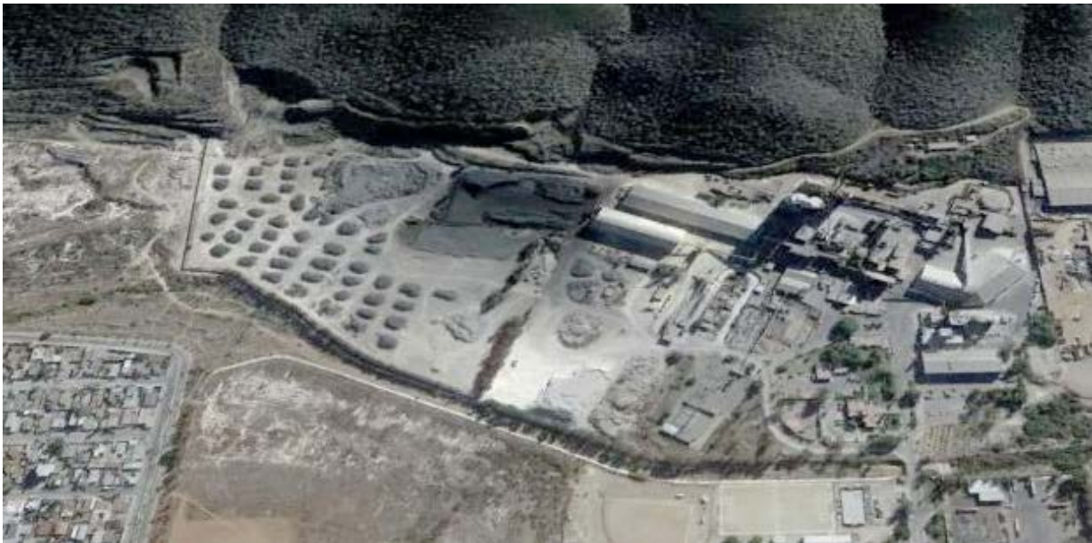
Image 13. Ensenada CEMEX plant with cells of waste tires, November 2016. Source: GoogleEarth.
