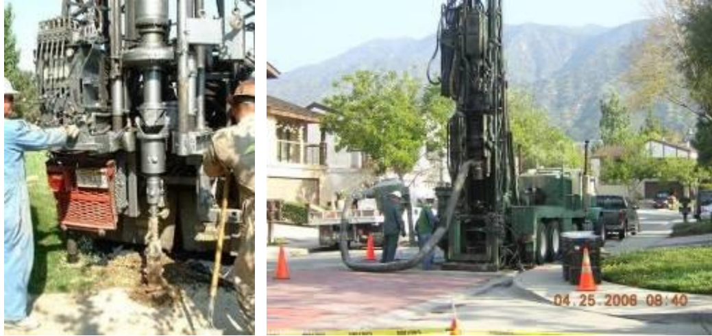
Figure 14: Drilling Equipment for exploration and sampling and gas monitoring well construction. Depending on geology and landfill materials a hollow-stem auger may suffice or site conditions may dictate the use of an air rotary or air-percussion drill rig; a local drilling company or geologist familiar with well installation in the area should be consulted
