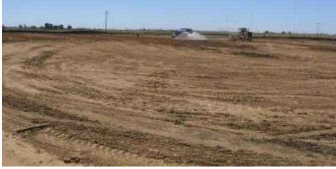
Figure 40: Remedial Cap Construction
