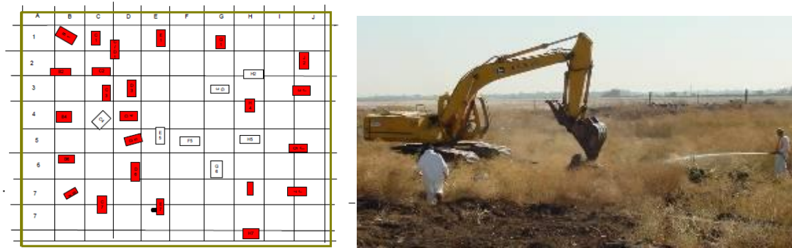
Figure 38: Trench Location Map; Trench Excavation & Dust Suppression
