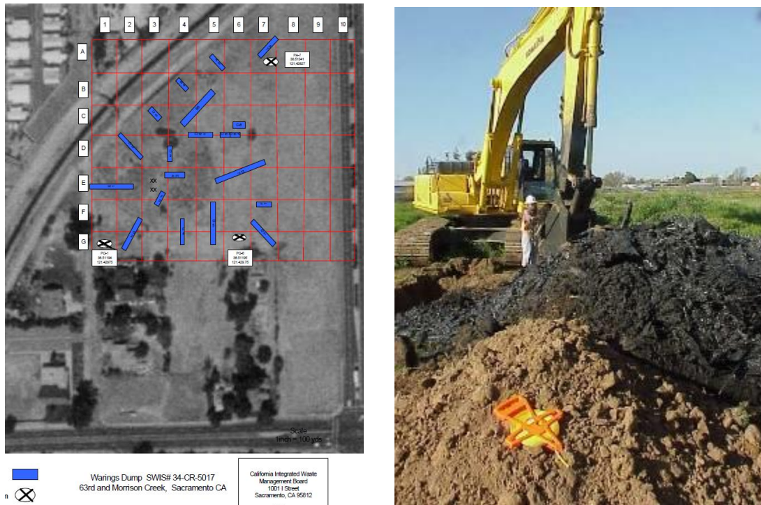
Figure 41: Trench Location Map; Trenching using a tracked excavator
