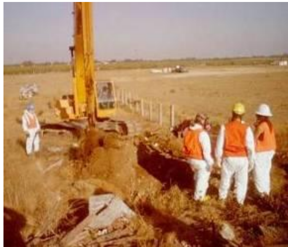
Figure 24: Sante Fe Road Sample Location Map depicting trenching and sampling locations to determine the waste extents and characteristics. Tracked Hoe or Excavator is used to perform trenching through cover, waste and native soils. Trenching provides data on the thickness of cover, the depth of waste to native soils and the physical and chemical characteristics of waste at the site.
