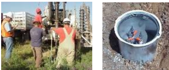
Figure 22: Drilling and Logging Gas Monitoring Wells. Completed Well Head Vault.
