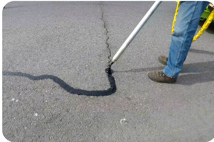
Figure 43. Crack sealing.
