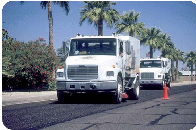
Figure 57. Sweeping loose aggregate.
