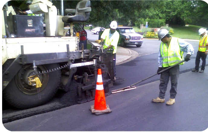
Figure 51. Raking and handwork.
