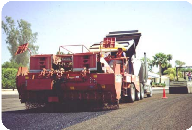
Figure 5. Applying aggregate.
