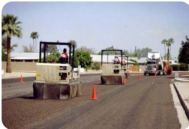
Figure 6. Rolling to embed aggregate.
