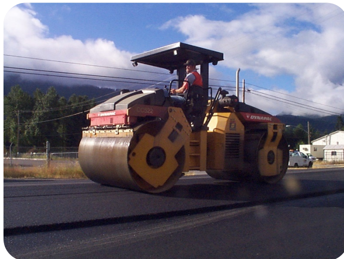
Figure 59. Steel-wheel roller.
