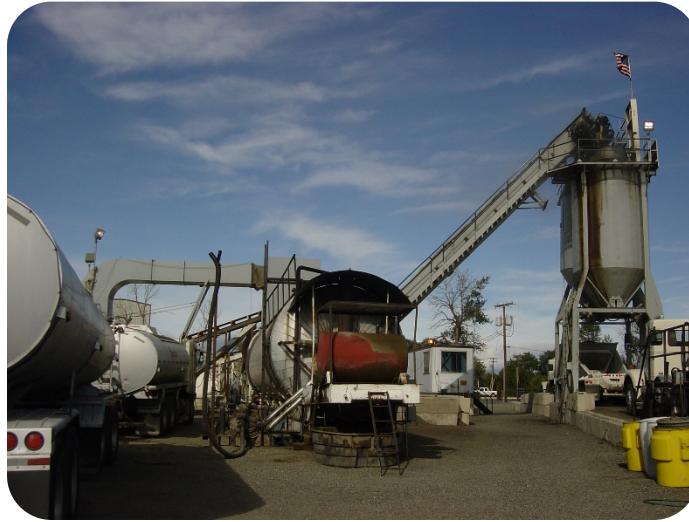
Figure 31. Asphalt binder storage tanks.
