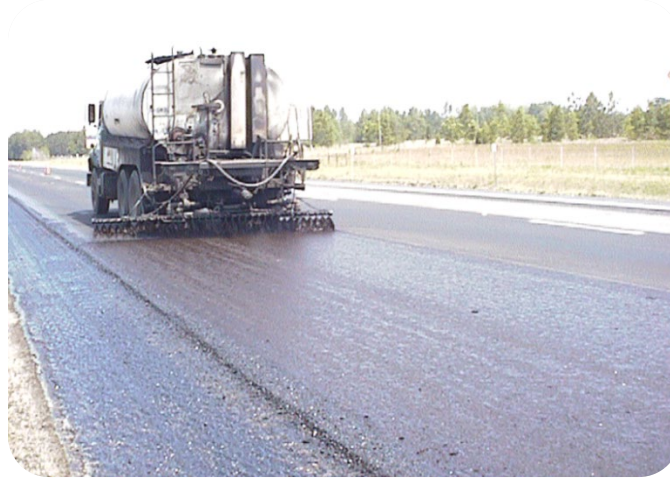
Figure 45. Tack coat distributor.
