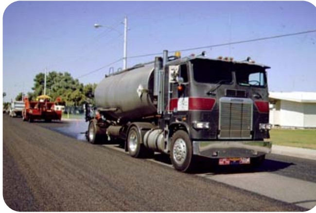
Figure 4. Spray application of binder.
