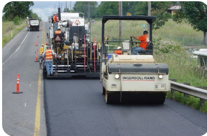
Figure 52. Roller compaction.
