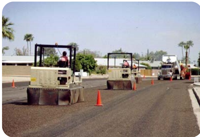
Figure 56. Rolling to embed aggregate into binder.
