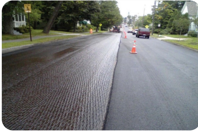
Figure 46. Uniform tack coat application.
