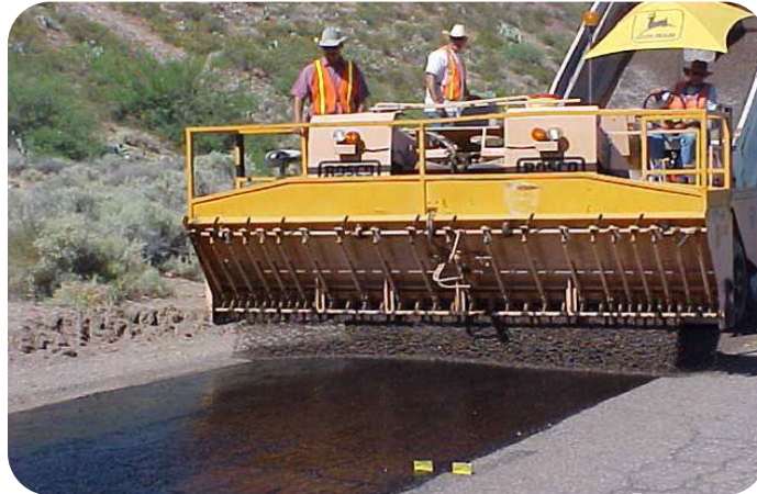
Figure 55. Aggregate spreader.
