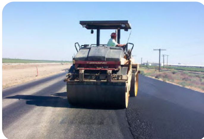
Figure 42. Use of steel wheel rollers.
