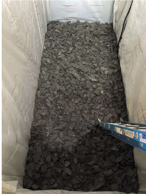
Figure 6.11 Placement of TDA.
