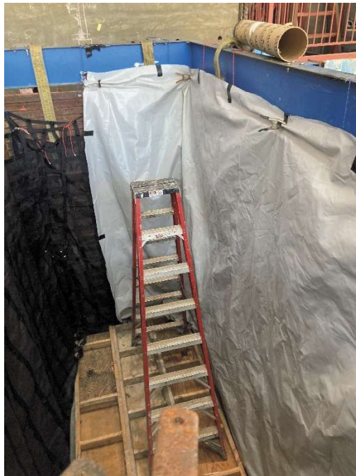
Figure 6.10 Installation of cargo nets and visqueen plastic.
