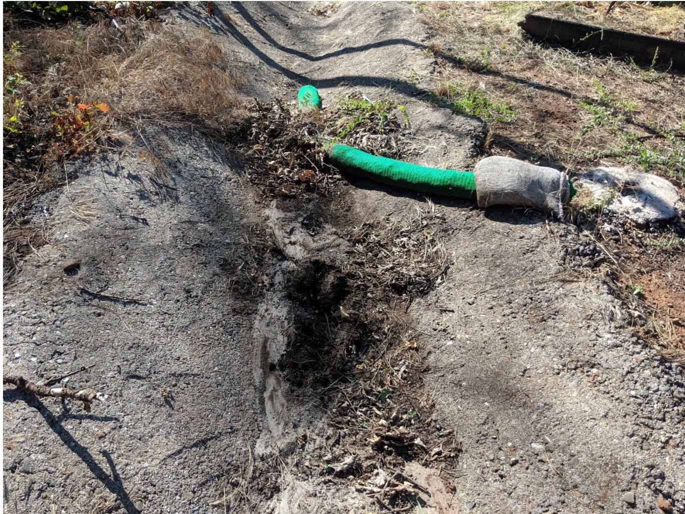
Figure 19: Example of an improperly deployed compost filter sock after the Camp Fire. Photo credit: Jackson Webster.
