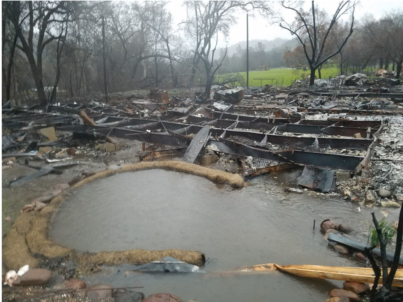
Figure 18: Another example of an improperly deployed and maintained straw wattle after the Camp Fire. Photo credit: Jackson Webster.
