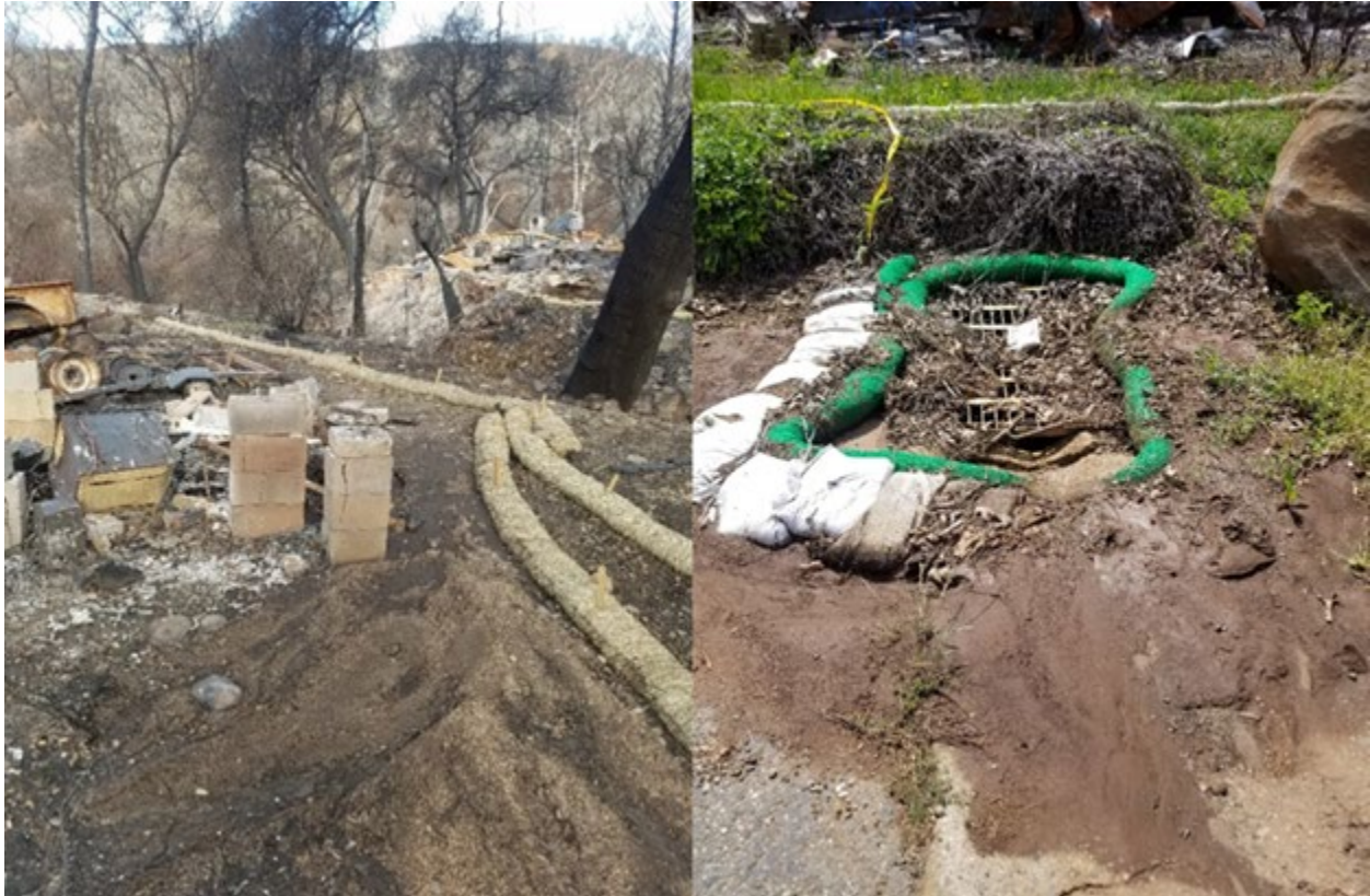
Figure 1A: Example placements of SW (left) and CFS (right) following the Camp Fire. Photo credits: Jackson Webster (left) and Sandrine Matiassek (right).
