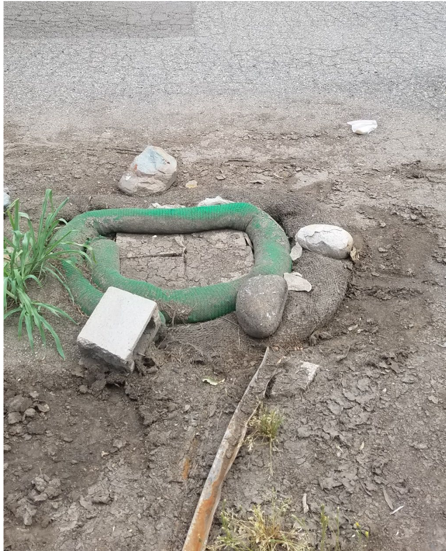
Figure 20: Example of improperly deployed straw wattle after the Camp Fire. Photo credit: Jackson Webster.
