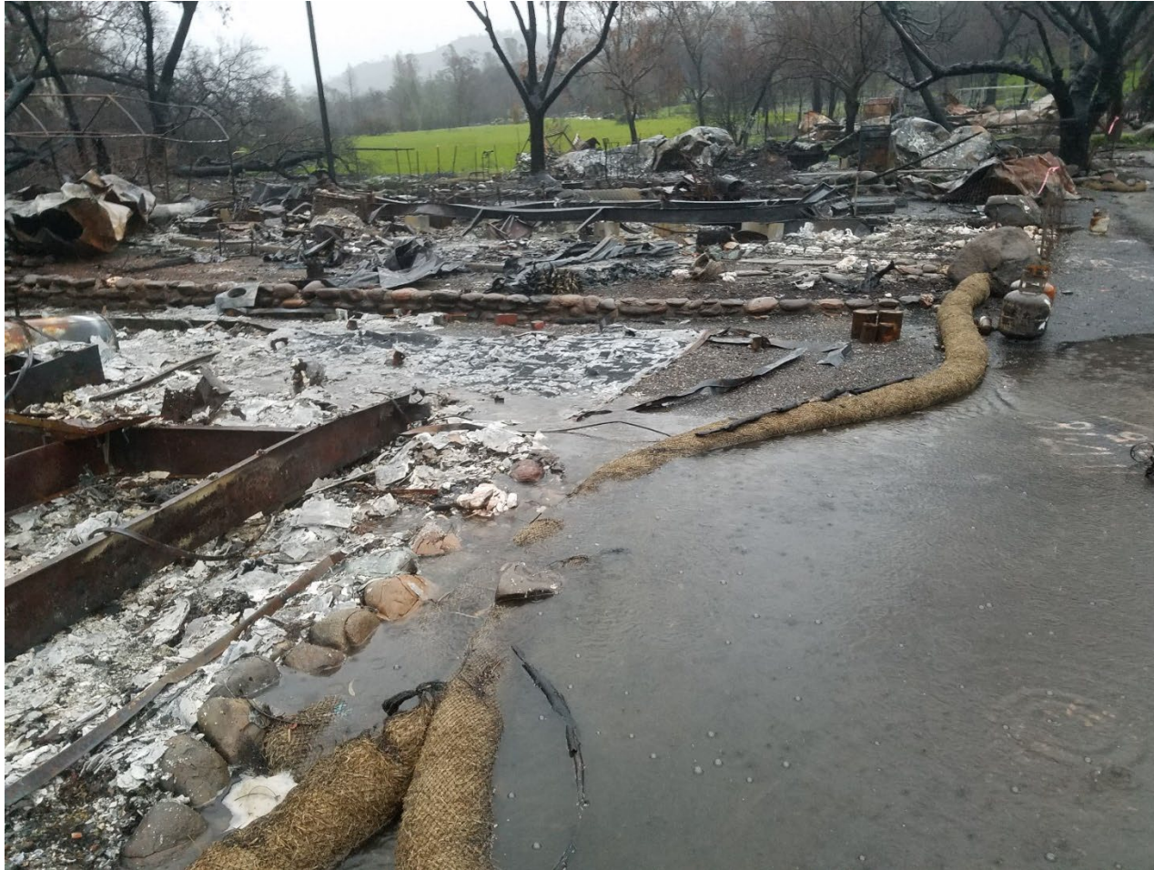
Figure 17: Example of an improperly deployed and maintained straw wattle at a mobile home park burned by the Camp Fire. Photo Credit: Jackson Webster.
