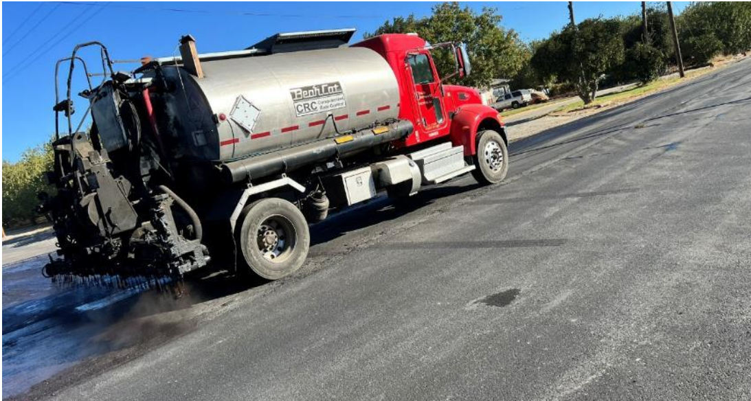
Figure 19. Tack coat application
