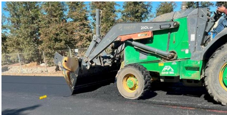
Figure 23. Loader cutting stop and start transitions for each material
