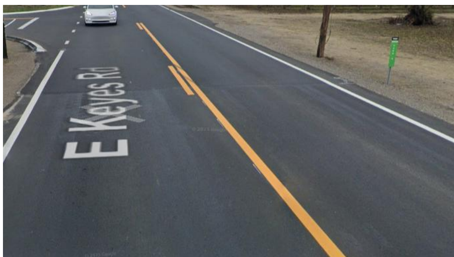
Figure 24. Transition between PelletPAVE-TR and HMA (courtesy Google Streetview)
