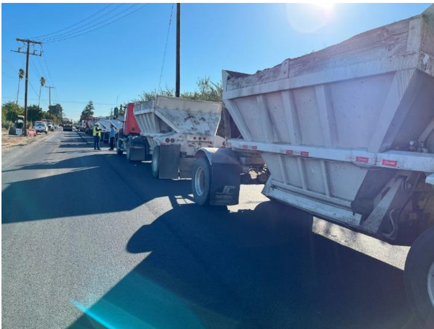
Figure 17. Mix delivery truck staging on East Keyes Road
