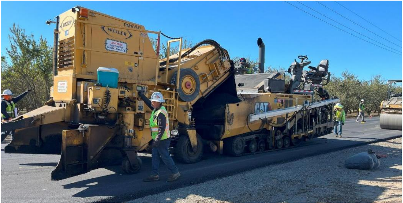
Figure 21. Pickup machine and paver staged for next material
