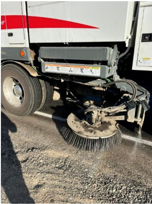
Figure 18. Initial brooming of pavement
