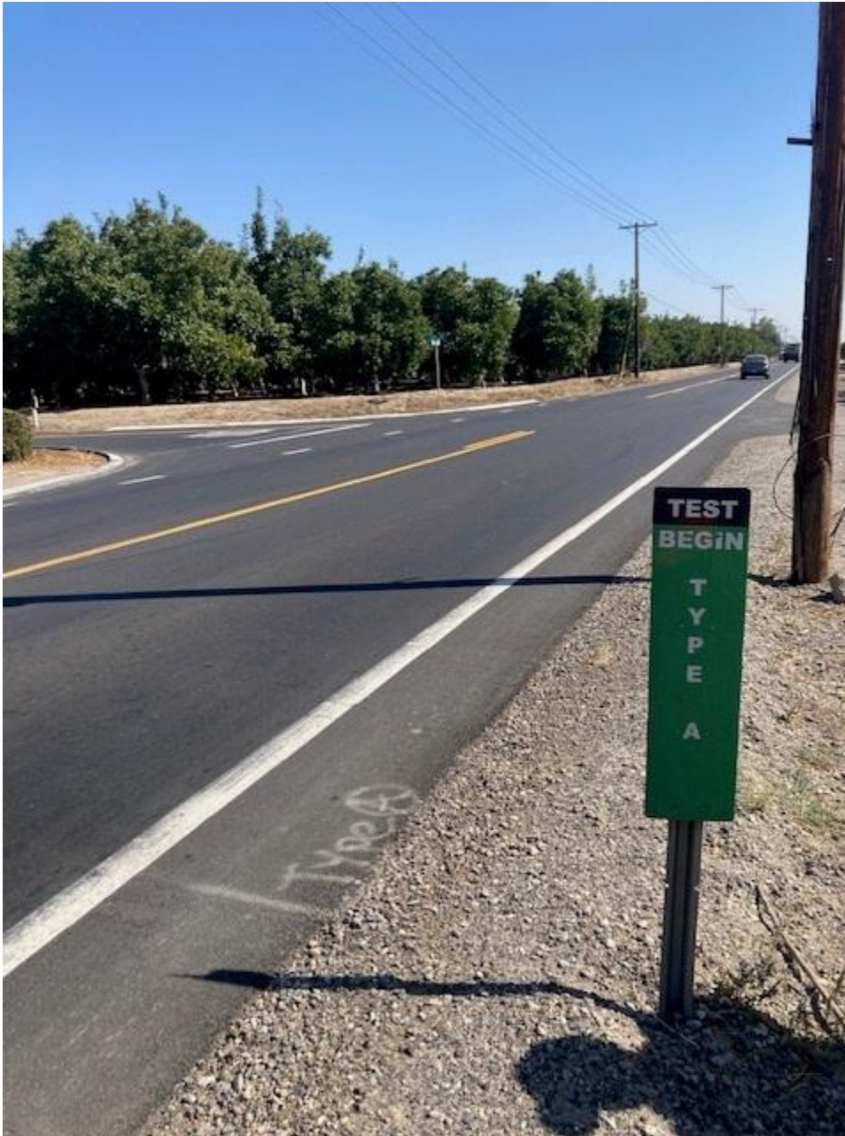
Figure 30. Beginning of conventional HMA test section October 2025
