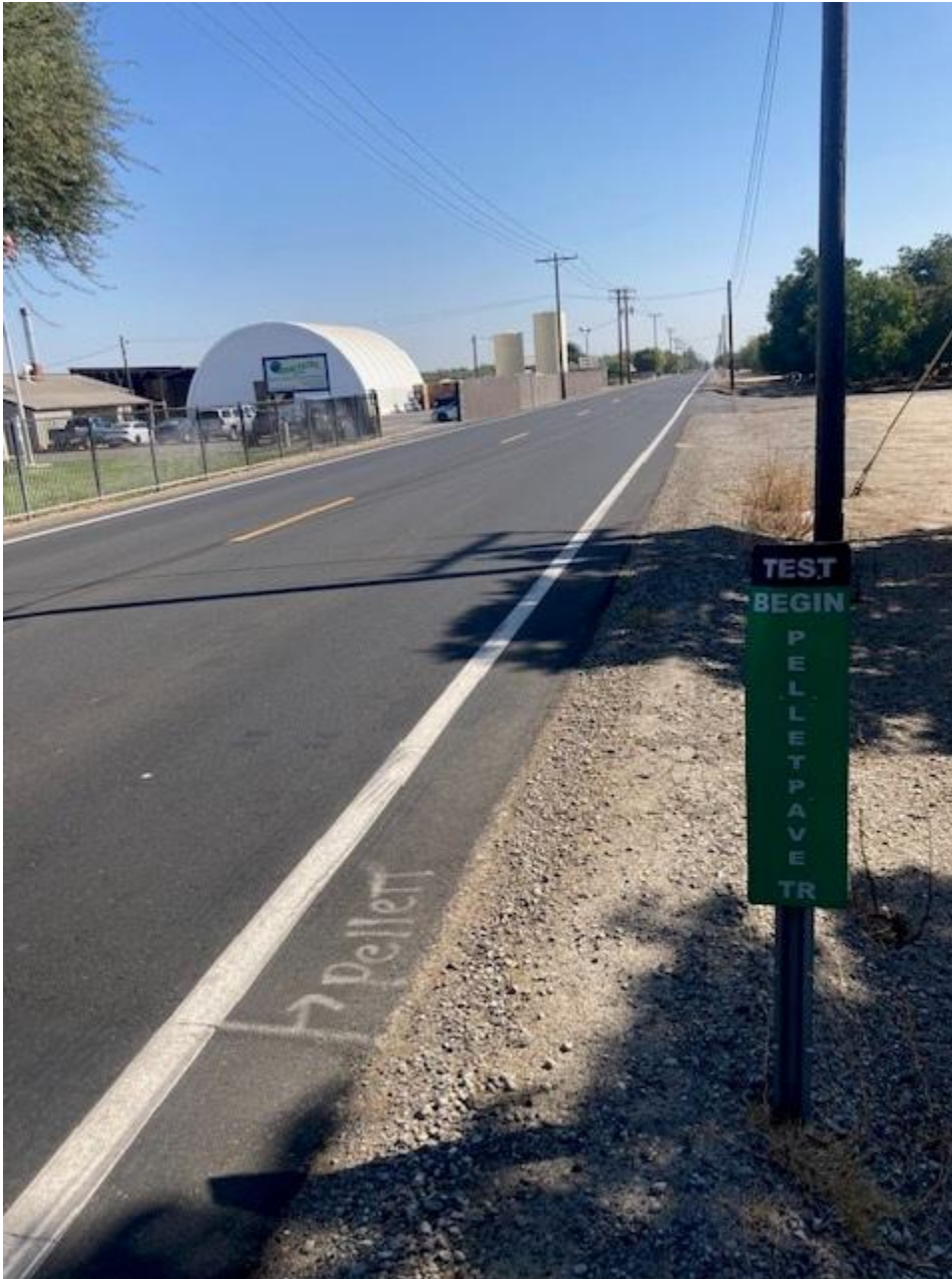
Figure 29. Beginning of PelletPAVE-TR test section October 2025
