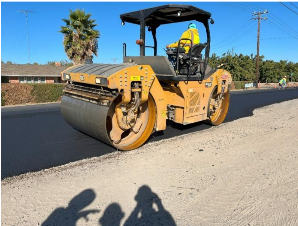
Figure 22. Compaction rolling
