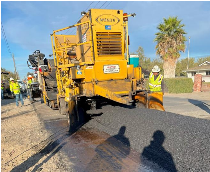
Figure 20. Windrow and pickup machine
