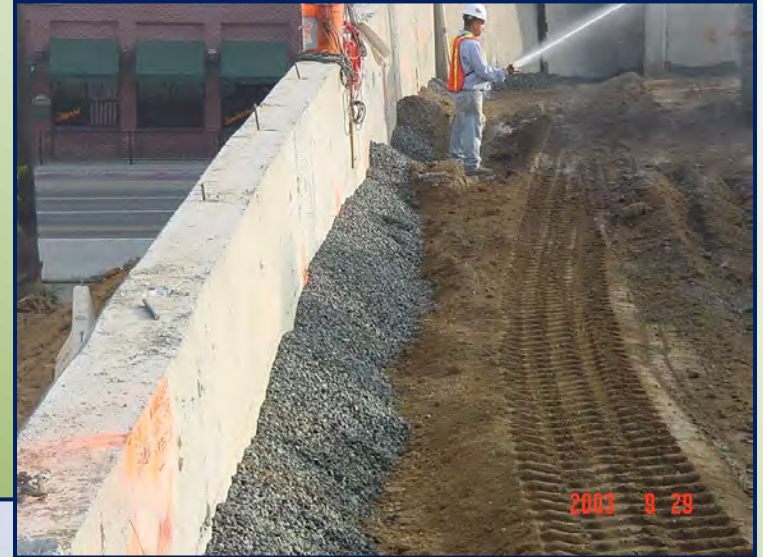
Typical gravel/soil section
