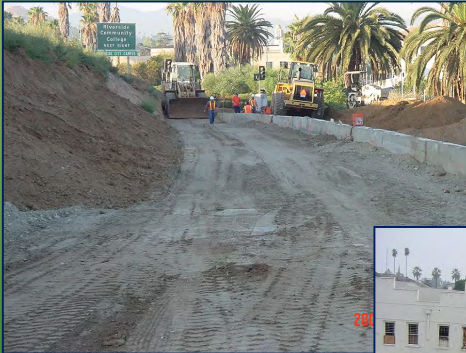
Completed cover soil installation, 2 feet
