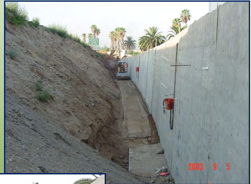
Compaction of foundation soil
