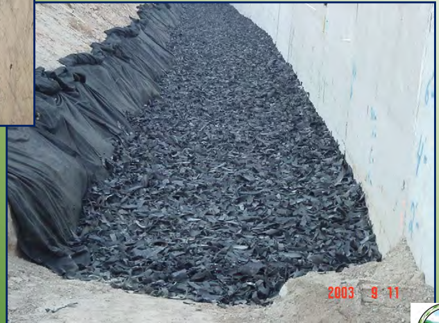
TDA placed and compacted
