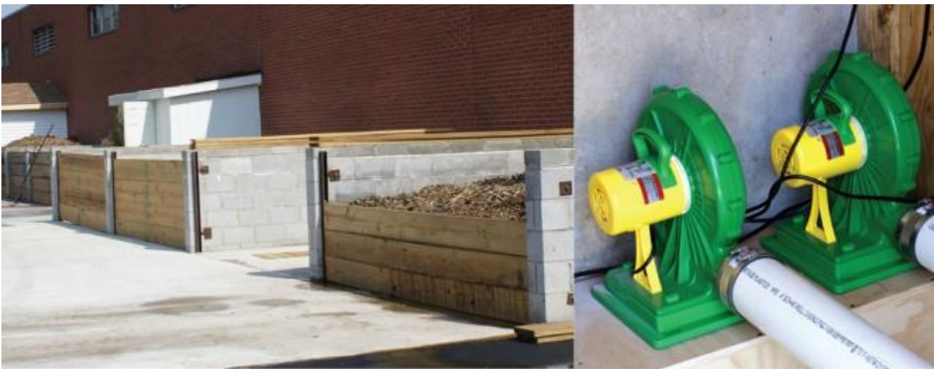
Food scraps and wood chips are composted in aerated bays (left) designed by O2Compost. Several low horsepower fans (right) service multiple bays.
