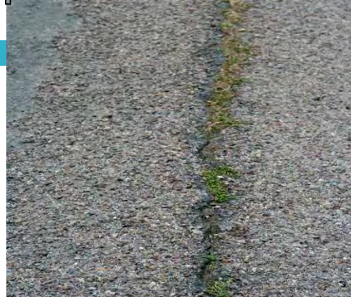
Longitudinal or transverse cracking
