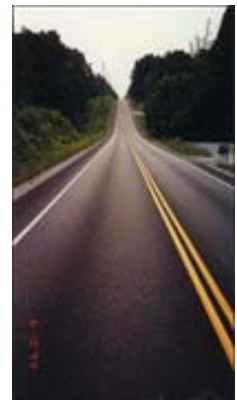
Hot mix asphalt Gap graded application
