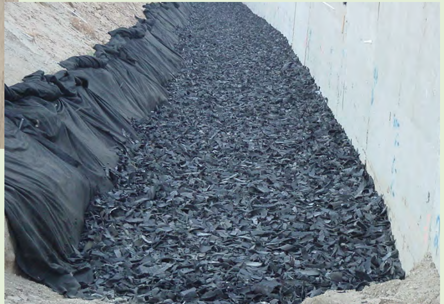
TDA placed and compacted
