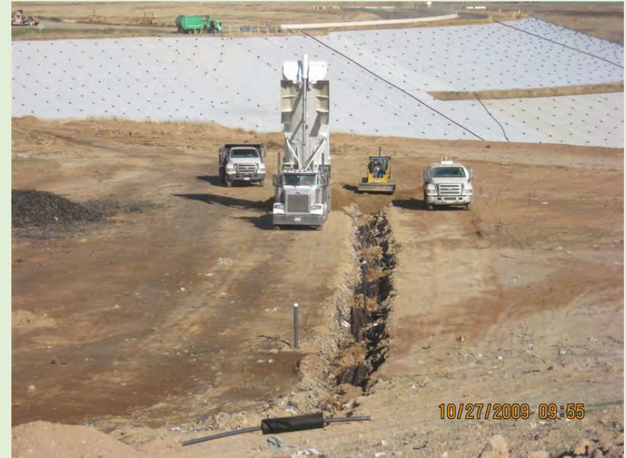
Kiefer Landfill, Leachate Recirculation and Gas Extraction trench design for Bioreactor landfill operation
