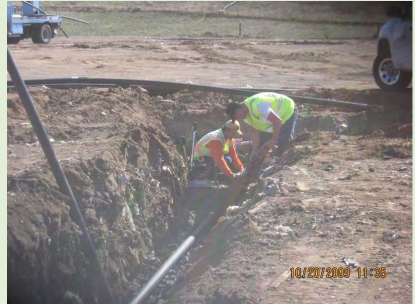
Welding of leachate injection pipe
