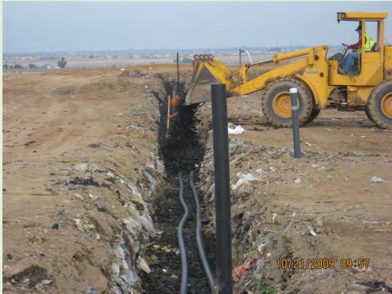
Trench extraction and recirculation lines installed
