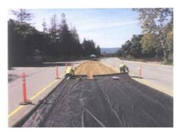
Photo Used: Preconstruction of the weed control fabric being placed before the rubber mulch (TDP) infill.
