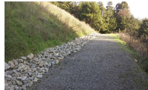
Fortuna Burn Dump After Remediation
