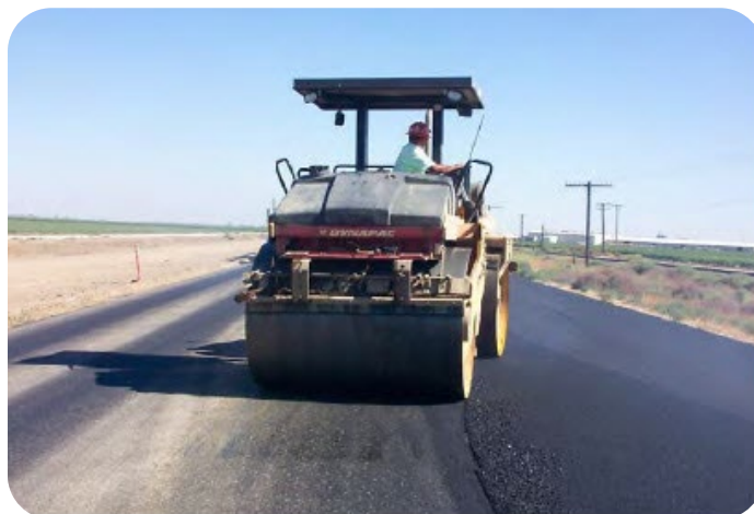
Figure 42. Use of steel wheel rollers.
