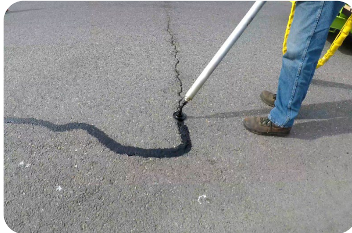
Figure 43. Crack sealing.
