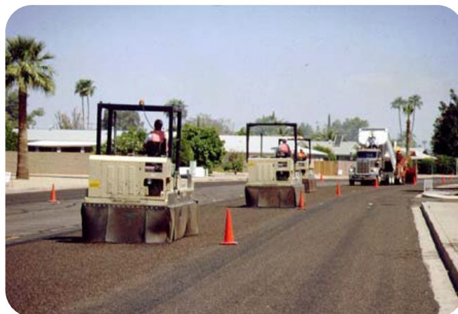
Figure 6. Rolling to embed aggregate.
