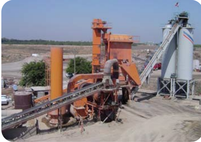
Figure 36. Hot mix asphalt plant.
