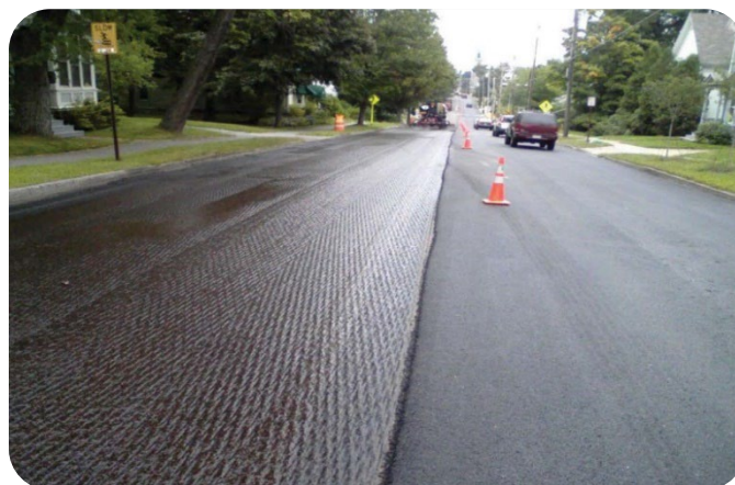
Figure 46. Uniform tack coat application.
