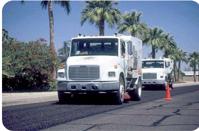
Figure 57. Sweeping loose aggregate.
