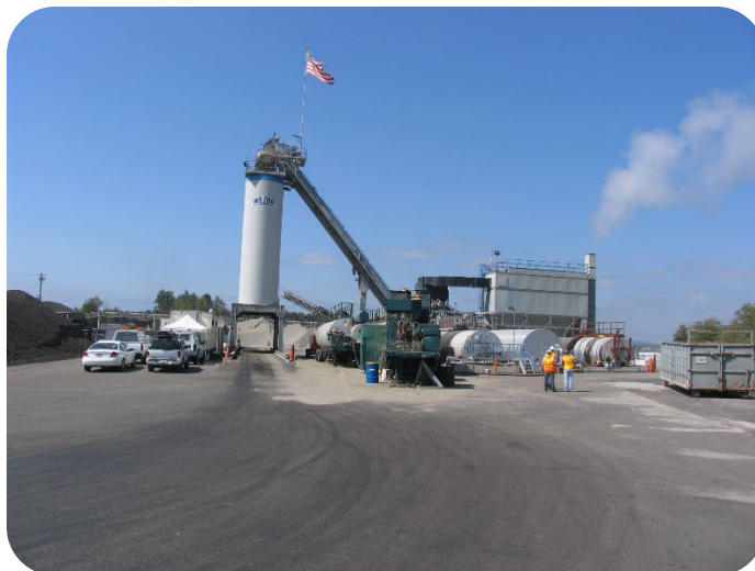
Figure 34. Asphalt rubber binder production.
