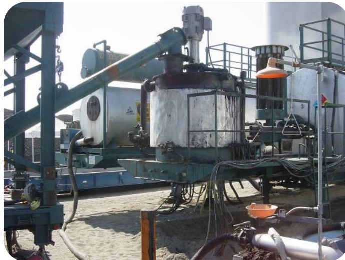
Figure 33. Feeding and blending equipment.
