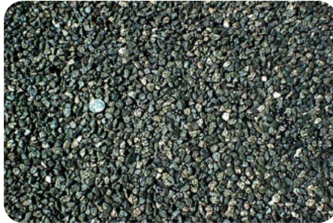
Figure 7. Finished chip seal surface.
