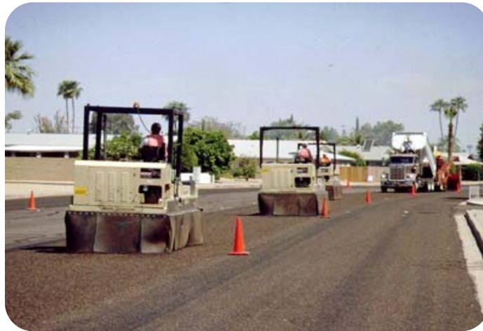
Figure 56. Rolling to embed aggregate into binder.
