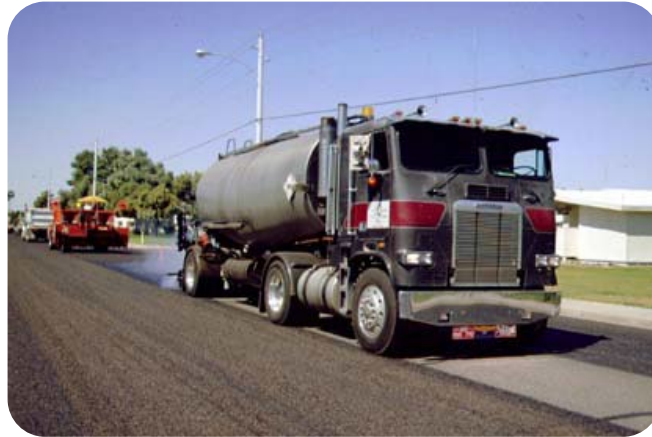
Figure 4. Spray application of binder.
