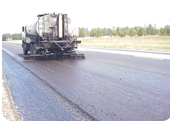
Figure 45. Tack coat distributor.
