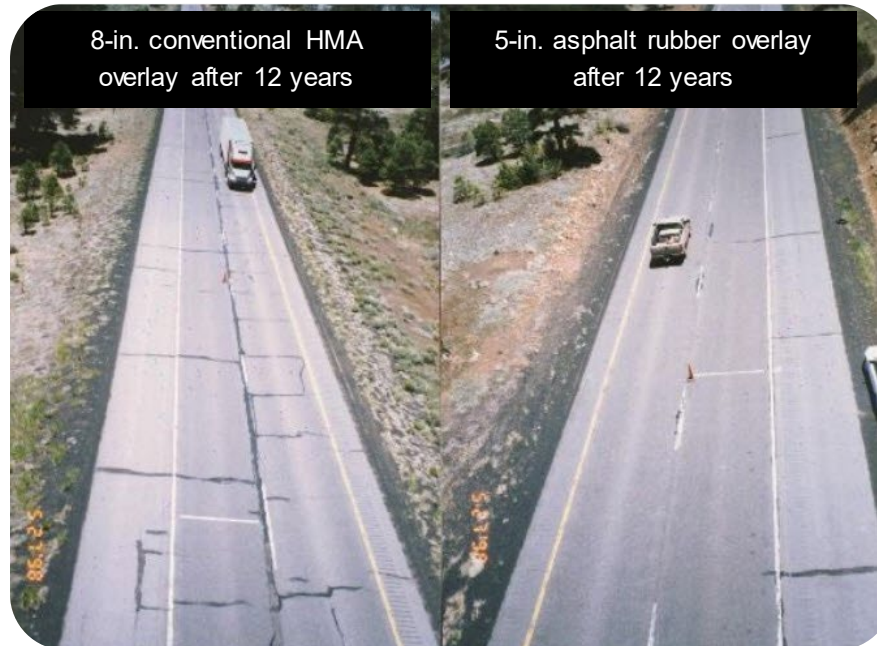
Figure 20. Asphalt rubber interlayers.
