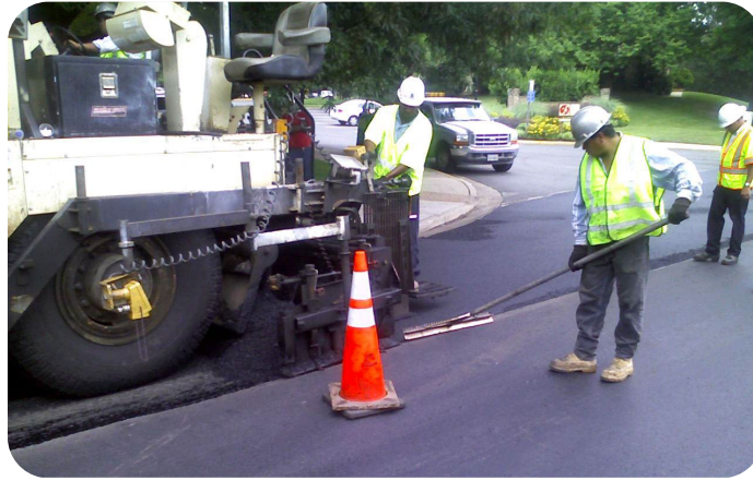
Figure 51. Raking and handwork.
