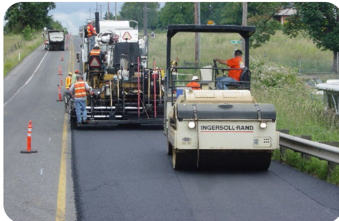
Figure 52. Roller compaction.
