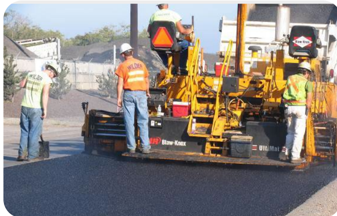
Figure 50. Mix placement.
