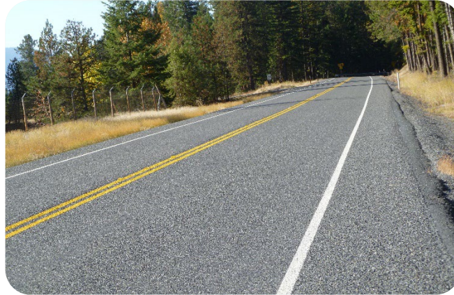
Figure 17. Chip sealed roadway.
