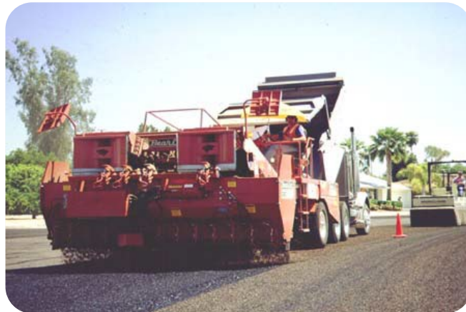
Figure 5. Applying aggregate.
