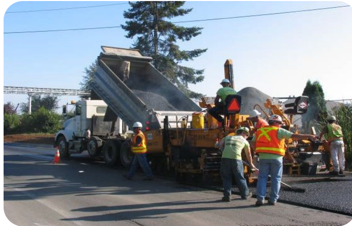
Figure 47. Delivery of asphalt mix using end dump truck.
