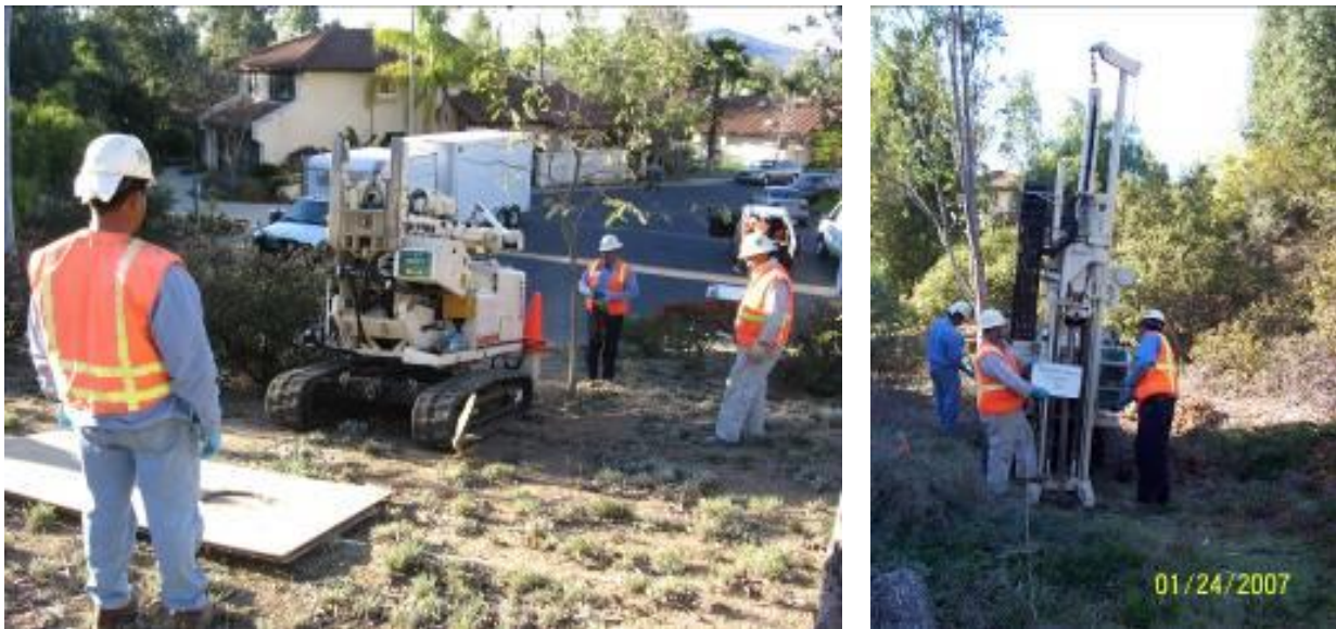
Figure 32: Small-tracked Hydraulic Direct-Push Rig used for intrusive investigation due to terrain and limited vehicle access
