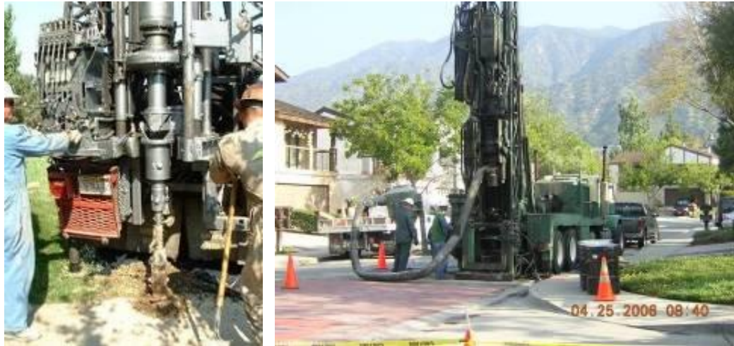
Figure 14: Drilling Equipment for exploration and sampling and gas monitoring well construction. Depending on geology and landfill materials a hollow-stem auger may suffice or site conditions may dictate the use of an air rotary or air-percussion drill rig; a local drilling company or geologist familiar with well installation in the area should be consulted
