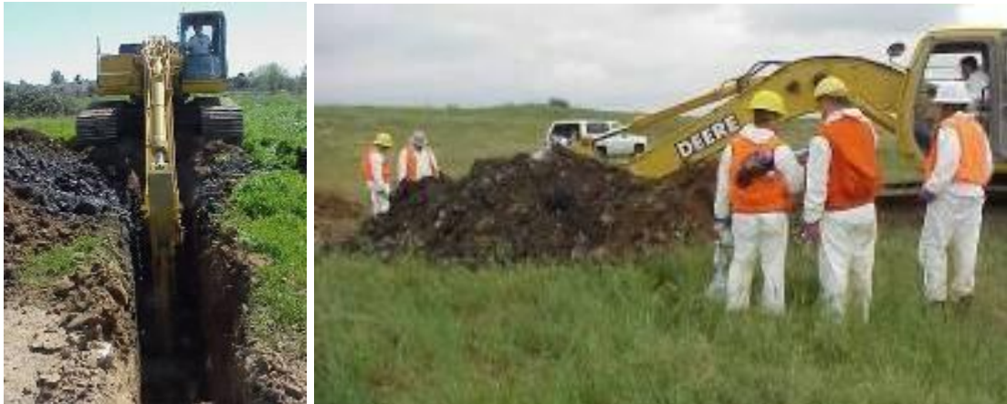
Figure 13: Trenching Investigation with a tracked-backhoe for Investigating Fills 15-25 feet in depth
