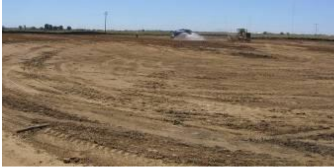
Figure 40: Remedial Cap Construction
