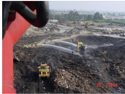
Figure 6. - C&D Disposal Site Fire
