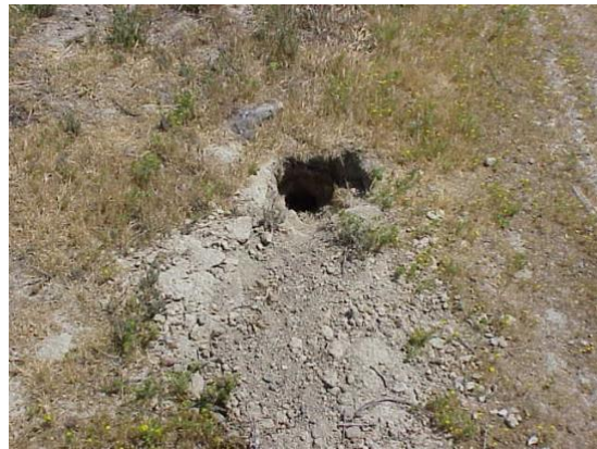
Figure 13 - Vectors damaging cover
