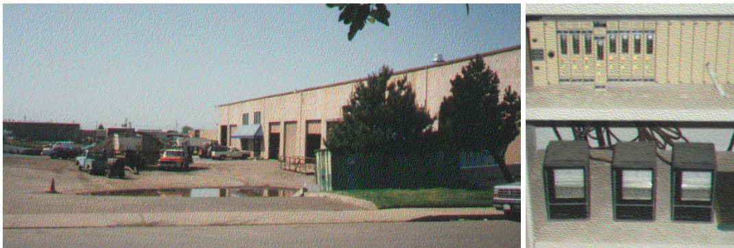
Figure 6: Sacramento Warehouse Constructed on a Former Landfill; Continuous Monitoring System
