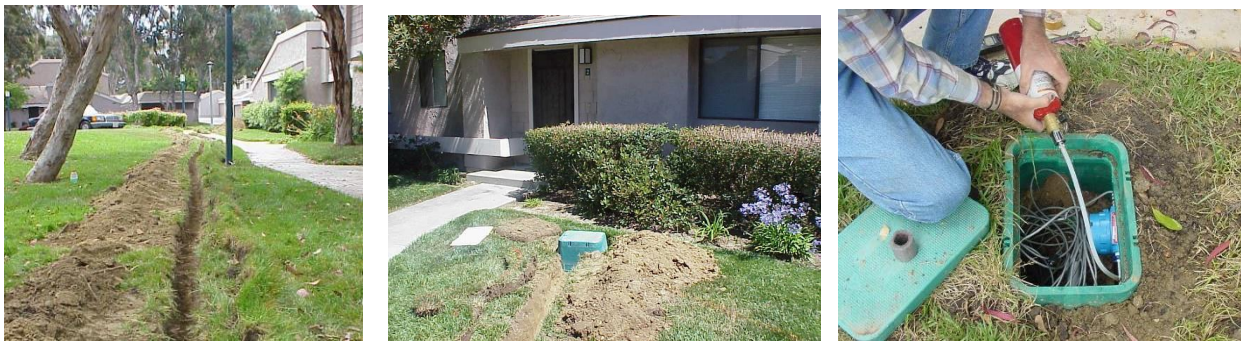
Figure 9: Trench for Sensor Cable; Sensor Vault adjacent to Condominium; Sensor Calibration
