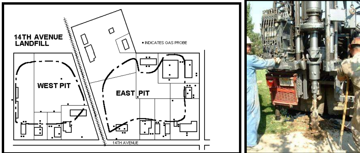
Figure 47: 14 th Avenue Landfill, Sacramento – Commercial development; installing a landfill gas well
