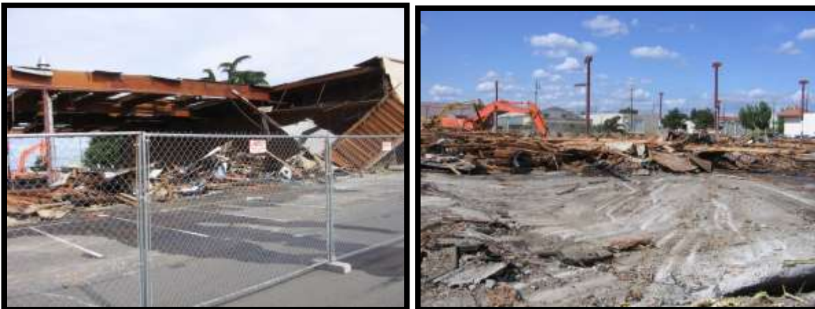
Figure 50: Commercial warehouse demolition in May 2011
