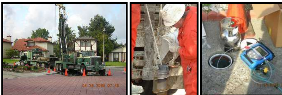
Figure 1: Constructing and monitoring landfill gas monitoring wells
