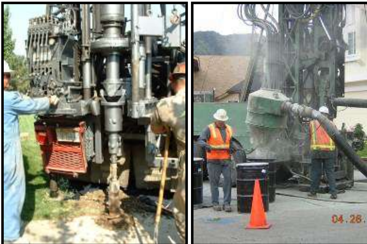
Figure 14: Drilling methods – hollow stem auger, air percussion
