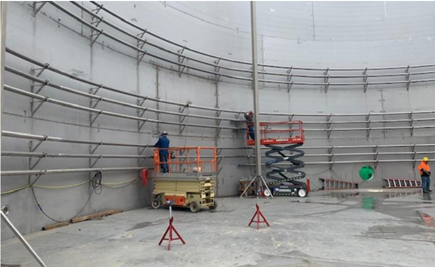
Rialto Bio- energy Facility, Rialto, CA
