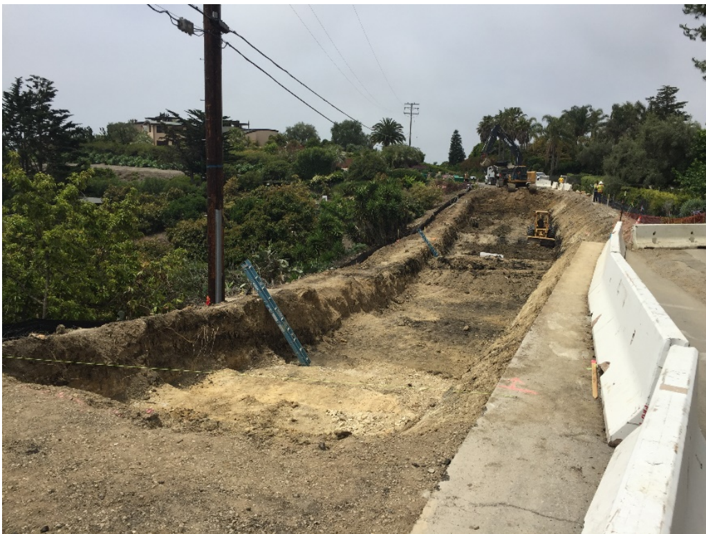
Figure 5.14: Excavation of the Failed Embankment Material
