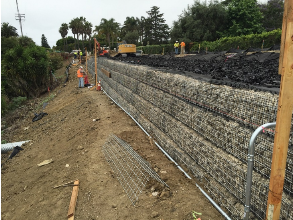
Figure 5.25: Placement of the Fourth Above-Ground TDA Lift and Checks on the Batter of the Gabion Wall Facing
