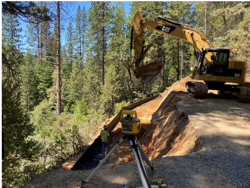
Figure 5.50: Initial Excavation and Placement of the First Welded Wire Mesh Reinforcement/Facing Unit
