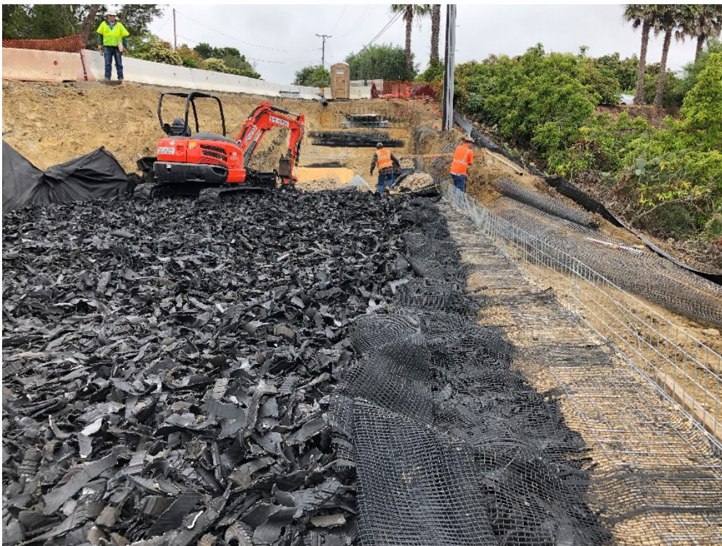
Figure 5.16: Placement of the First Above-Ground Gabion And Preparation of the Reinforcement layer to be stretched across the TDA
