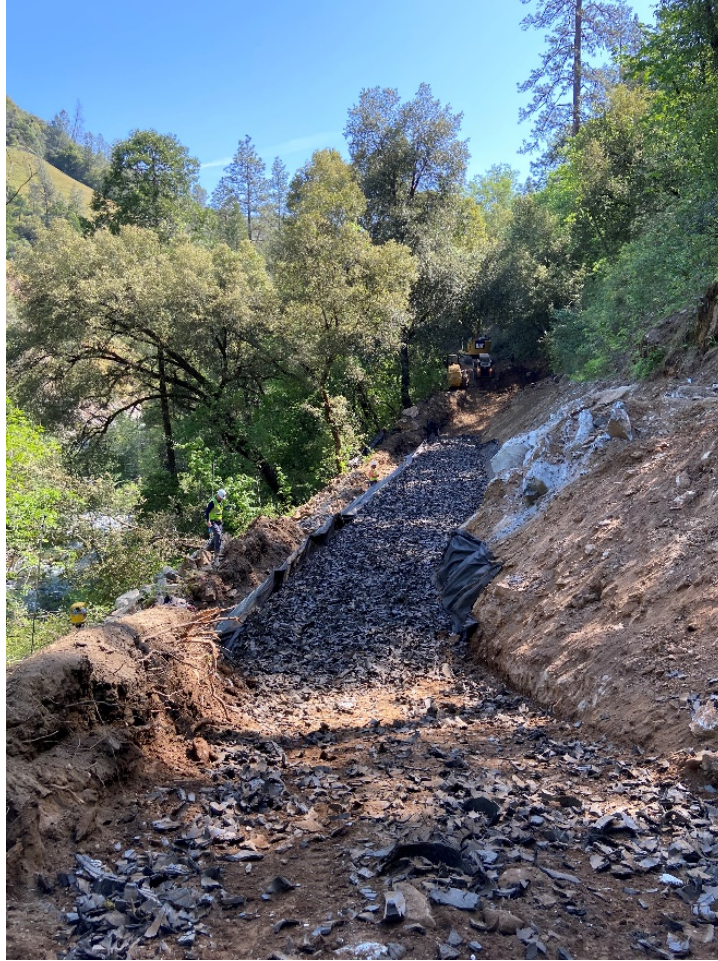
Figure 5.38: Placement of First Lift of TDA
