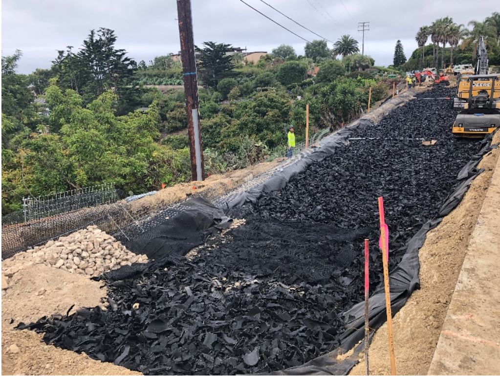
Figure 5.17: Placement of the Second Above-Ground TDA Lift
