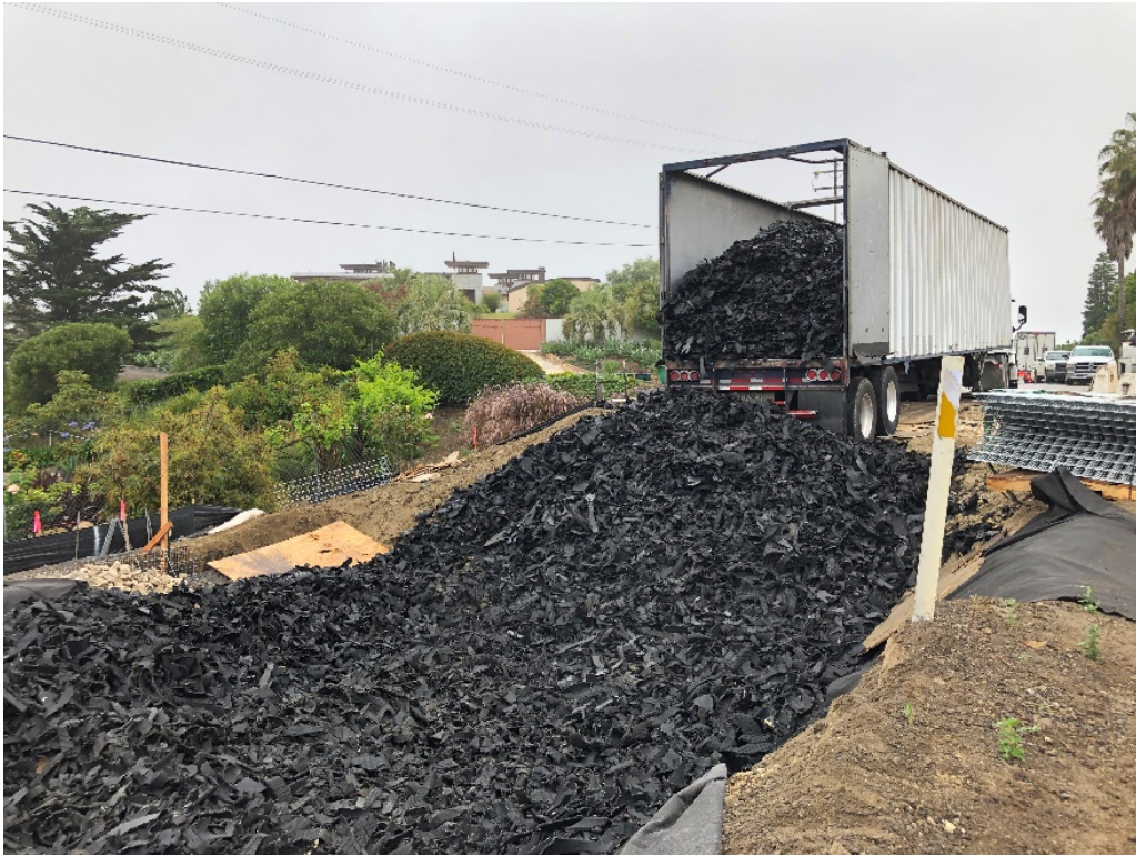
Figure 5.15: Placement of TDA Within the Excavation
