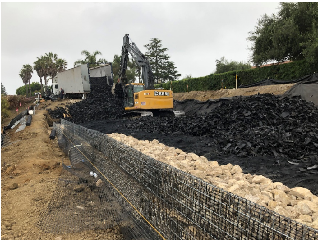
Figure 5.18: Picture Showing the Geosynthetic Wrapped Around the Facing while a TDA Lift Is Being Placed By an excavator
