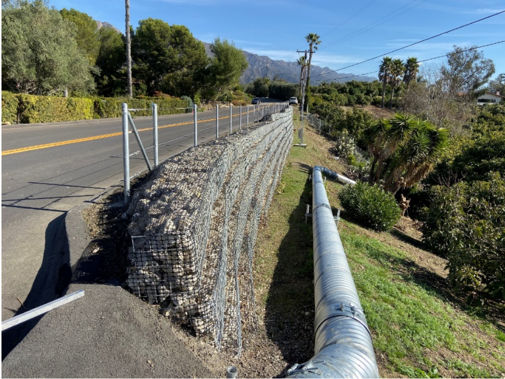
Figure 5.27: Final MSTDA Wall at Ortega Ridge Road from the South
