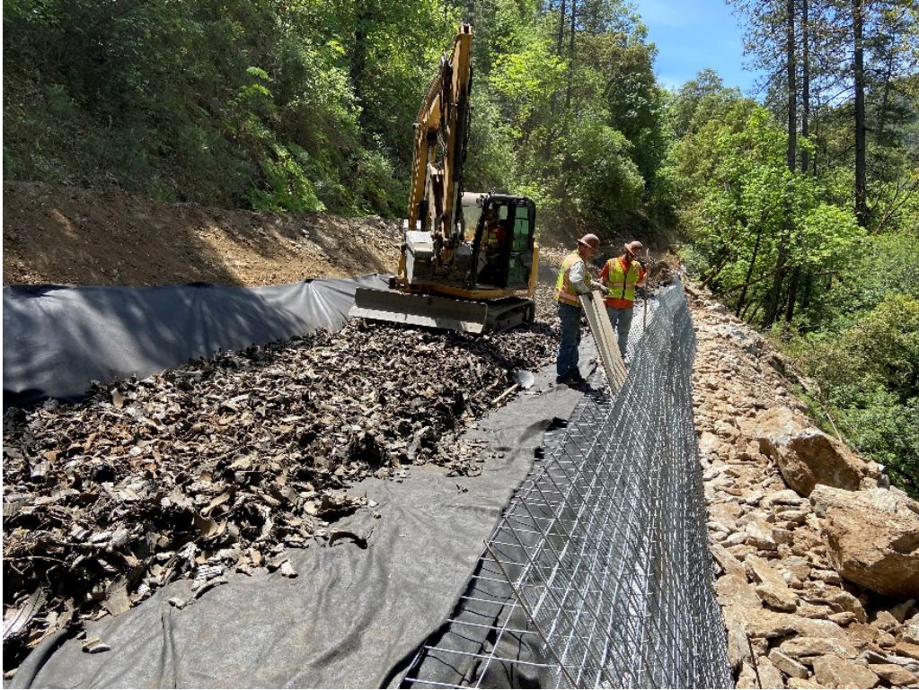
Figure 5.40: Placement of Third Lift of TDA
