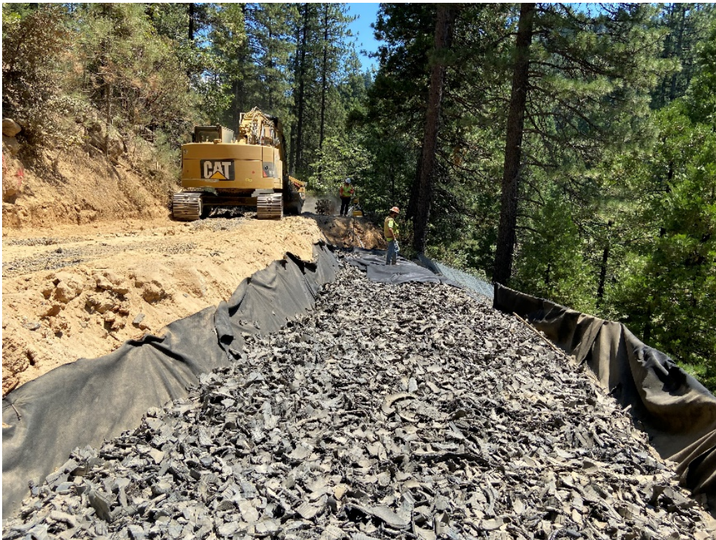
Figure 5.55: Placement of a TDA lift
