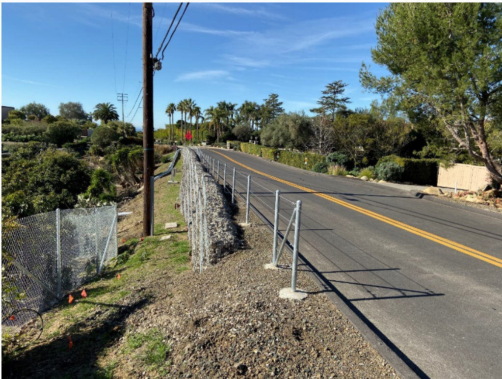
Figure 5.26: Final MSTDA Wall at Ortega Ridge Road from the North
