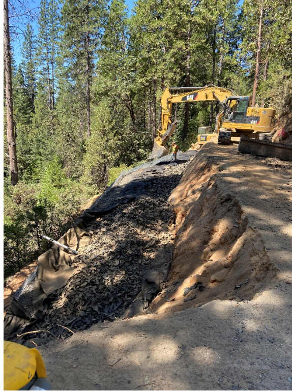
Figure 5.50: Placement of the First Lift of TDA
