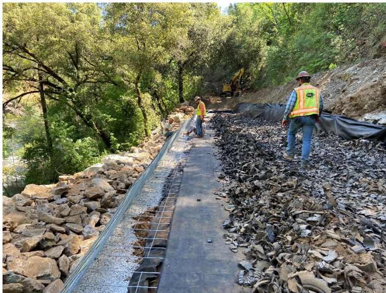
Figure 5.39: Facing Detail of the Metallic Hilfiker Mesh Layers, with Nonwoven Geotextile Atop Metallic Reinforcement
