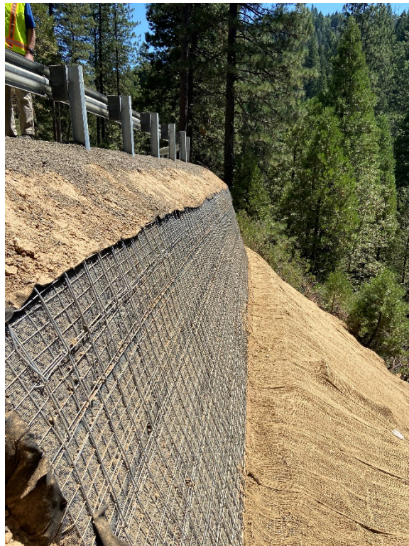
Figure 5.57: Final MSTDA Wall at Italian Bar Road Site 6 from South
