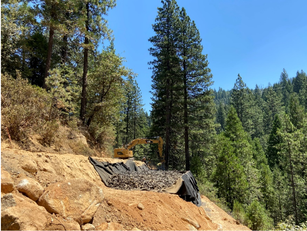
Figure 5.54: Placement of a TDA lift
