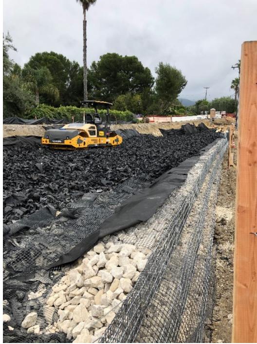
Figure 5.19: Photo Showing the Compaction of the TDA Using a Vibratory Sheepfoot Roller
