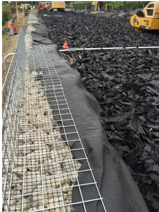
Figure 5.24: Picture of a Utility Line Running through the TDA Along with a Highlight of the Separator Geotextile Between the Crushed Rock and TDA, and the Biaxial Geogrid Placed Within the Gabions for Improved Retention of Rock Within the Gabions
