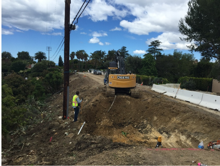
Figure 5.13: Initial Excavation of the Failed Embankment
