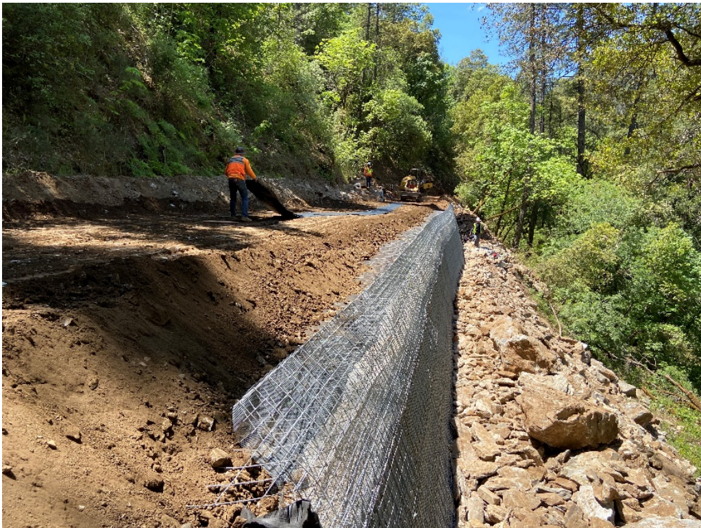
Figure 5.41: Placement of Granular Bearing Layer
