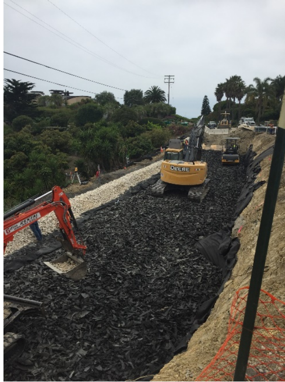
Figure 5.21: Placement of Crushed Rock into the Next Gabion Layer
