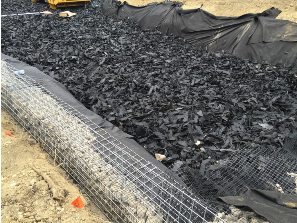
Figure 5.23: Preparation for Geogrid Placement at the Top of a TDA Lift
