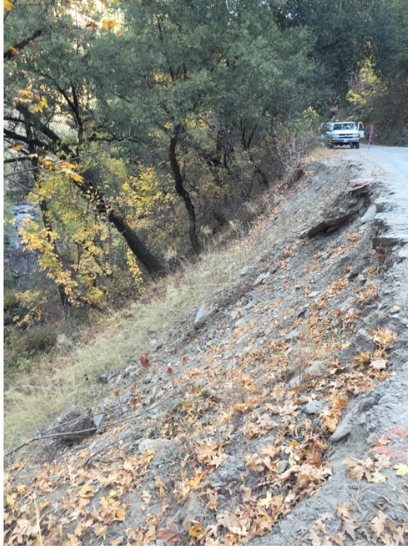
Figure 5.36: Italian Bar Road Site 3 Prior to Construction with Severe Shoulder Erosion
