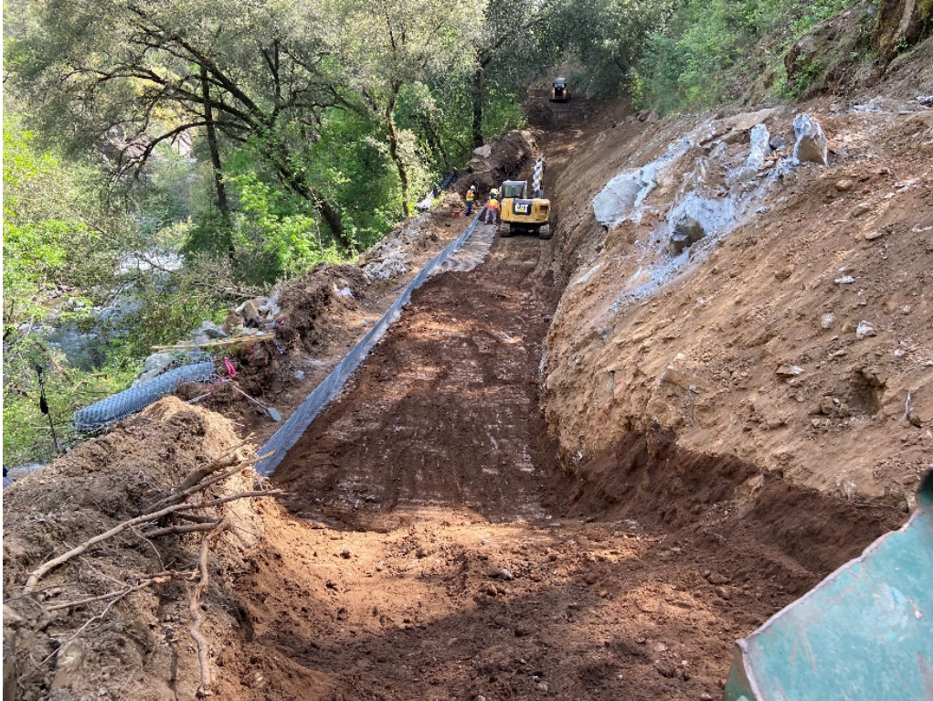
Figure 5.37: Excavation of the Existing Slope
