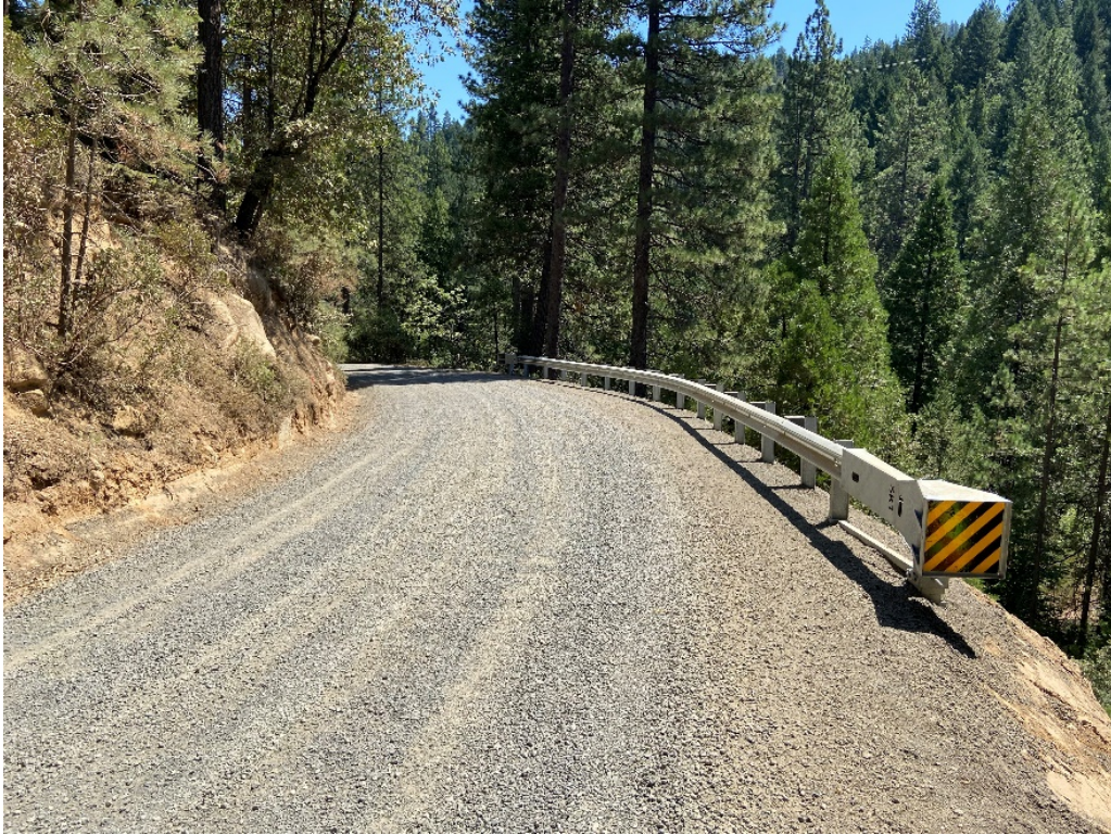
Figure 5.58: Final Unpaved Road atop the MSTDA Wall at Italian Bar Road Site 6 From South Showing Position of the Guard Rail in the Gravel Within the Top Gabion
