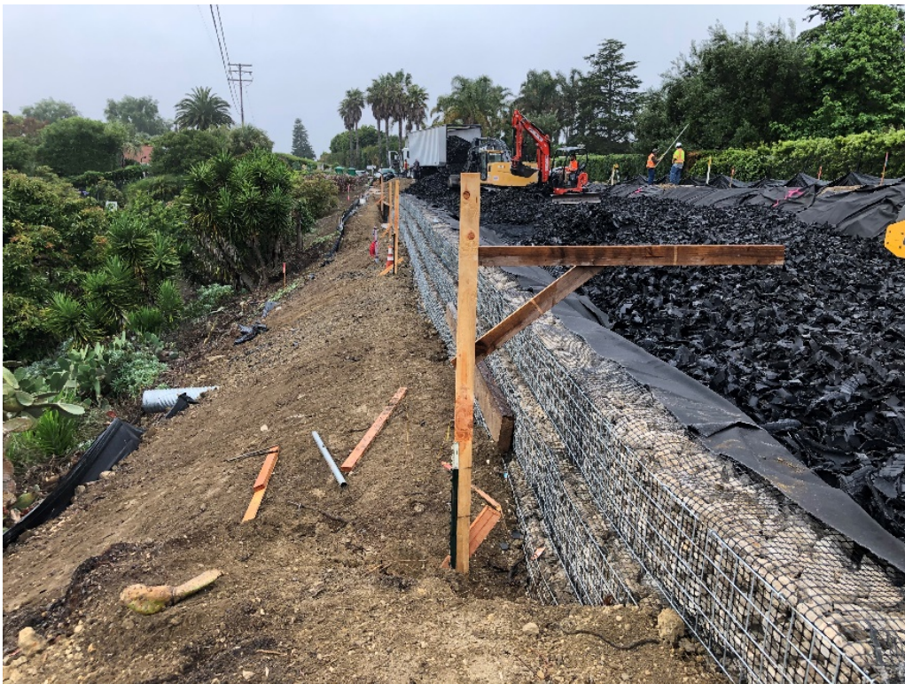
Figure 5.20: Picture of the Third Above-Ground TDA Lift Being Placed
