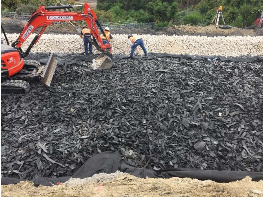
Figure 5.22: Picture of the Separator Geotextile Being Placed Between the Crushed Rock and TDA
