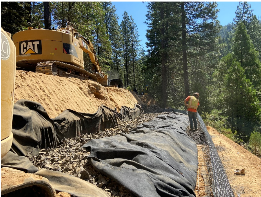
Figure 5.51: Encapsulation of TDA in Nonwoven Geotextile
