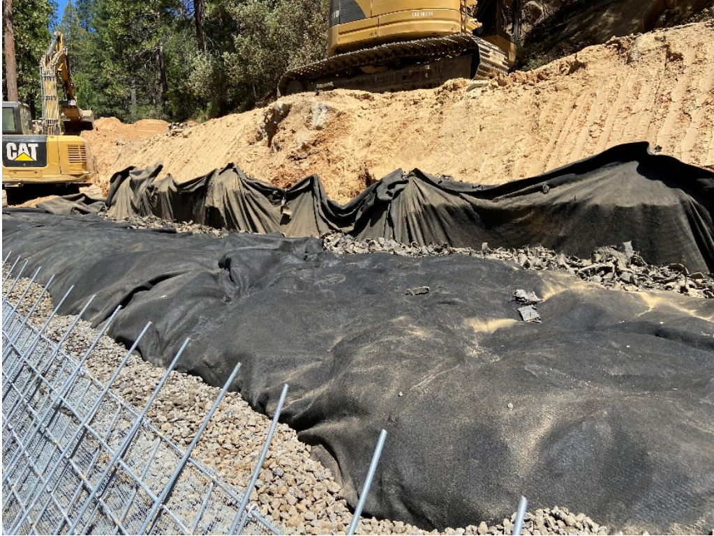
Figure 5.52: Placement of Gravel Near The Facing
