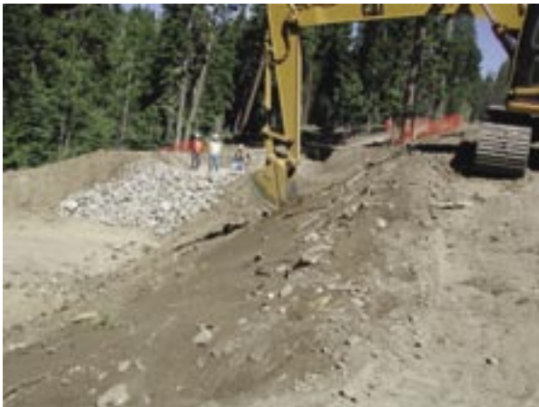
Compost incorporation, Placer County, Route 267. Photo courtesy of Caltrans
