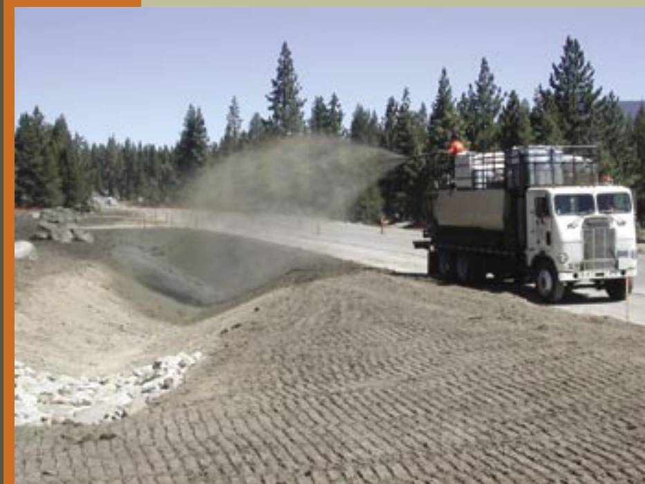
Compost and hydroseeding application. Photo Courtesy of Caltrans.
