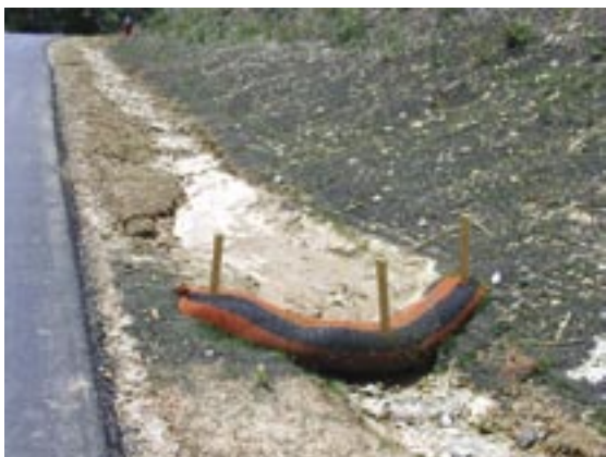
Filter sock, photo courtesy of Dr. Britt Faucette, Filtrexx
