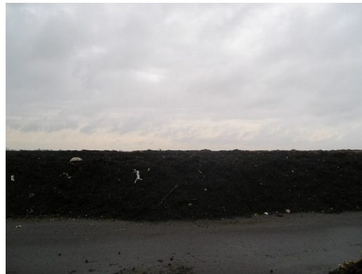
City of Chico Compost Facility
