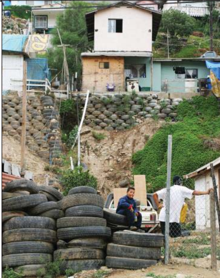
Plate 15. Scrap Tires in Tijuana Hillside Construction Throughout the city, there are many areas with intensive use of scrap tires for home construction and connecting stairways.
