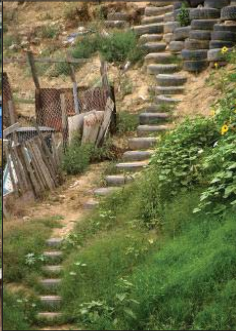
Plate 15. Scrap Tires in Tijuana Hillside Construction Throughout the city, there are many areas with intensive use of scrap tires for home construction and connecting stairways.
