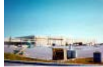
Parking Lots and Building
